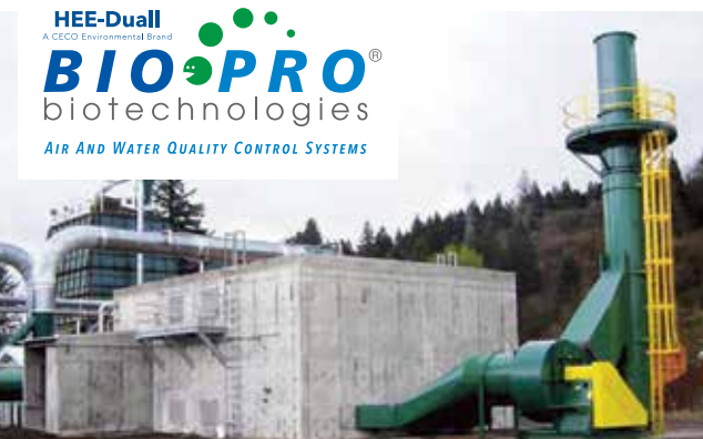
Biofilter Removing Hazardous Air Pollutants (HAPs)
