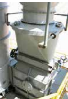
Venturi Scrubber System Treating Emissions from an Industrial Furnace
